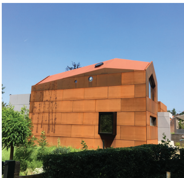
Architects' house - Belgium Terracotta roof surface combined with façade in Corten steel
