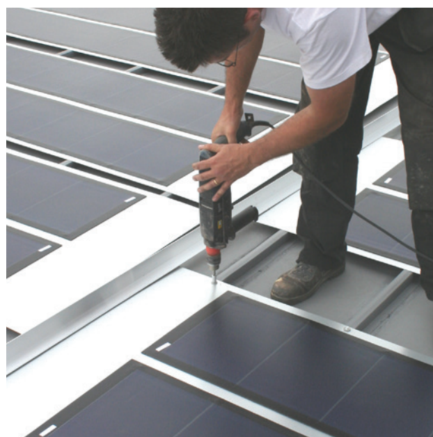
Replacing panels without the risk of damaging the roofing membrane.
